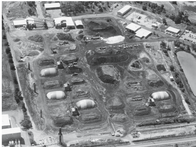
FIGURE 19.8 The Exolon plant in Hennepin, IL. This plant is one of the newest SiC facilities in the world, producing both high-quality metallurgical and crystalline SiC annually. It is North America's only manufacturer of SiC. The plant features 16 furnaces operating off of four transformers.
